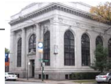
(FORMER) FULLERTON STATE BANK 1425 W. Fullerton Avenue Date: 1923 Architect: Karl M. Vitzthum
